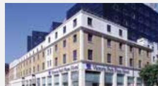
Park Plaza Victoria London Adjacent to Victoria Station
